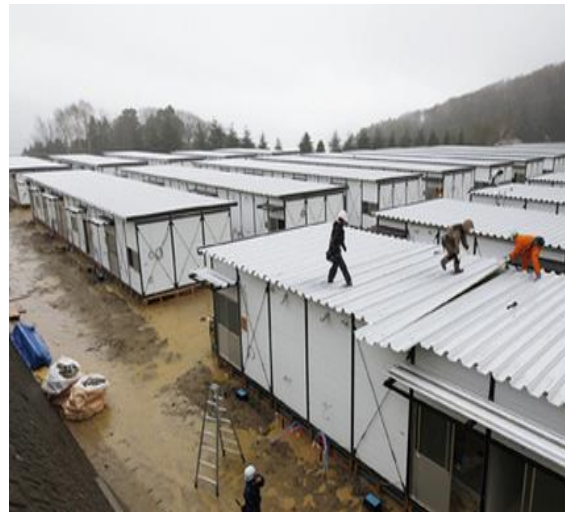
Pre-fabricated temporary houses with water supply and sewage treatment
