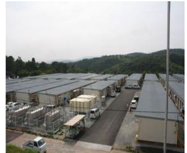
Pre-fabricated temporary houses with water supply and sewage treatment
