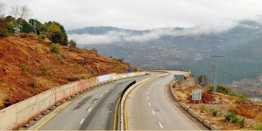
RCC Retaining Walls along Muzaffarabad-Islamabad Highway
