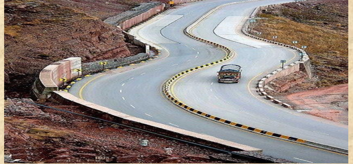
RCC Retaining Walls along Muzaffarabad-Islamabad Highway
